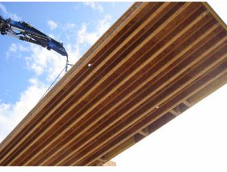
Crane lifting Home Technology's floor panel into place.
